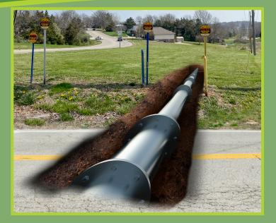
Pipeline markers and warning signs are used to indicate the presence of an underground pipeline right of way (ROW). Signs and markers must NOT be used or relied upon to determine the exact location of the underground utility. Always contact Missouri 811 for a locate before digging.
